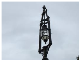
A Cause Celebre ! Heritage Lamposts- Victims Of Neglect Farncombe Road
