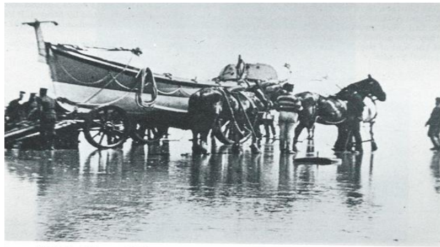
The Richard Coleman and his heavy transporting carriage on the sands, preparing to launch at low tide.
